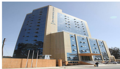
Project Name : Yotek Building Location : Addis Ababa
